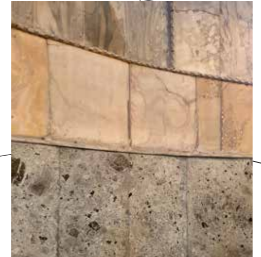
7. Athens, Greece Different final outcomes resulting from different processing methods applied to the same material from the same source.
